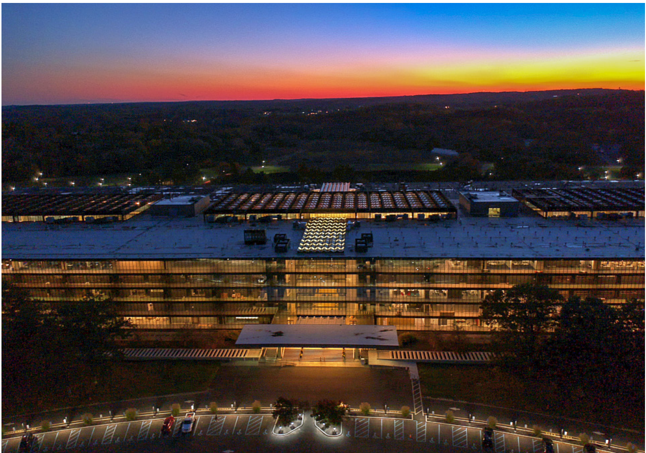
Bell Works - Holmdel, NJ
